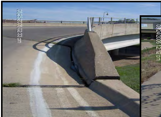
SIXTH STREET BRIDGE
